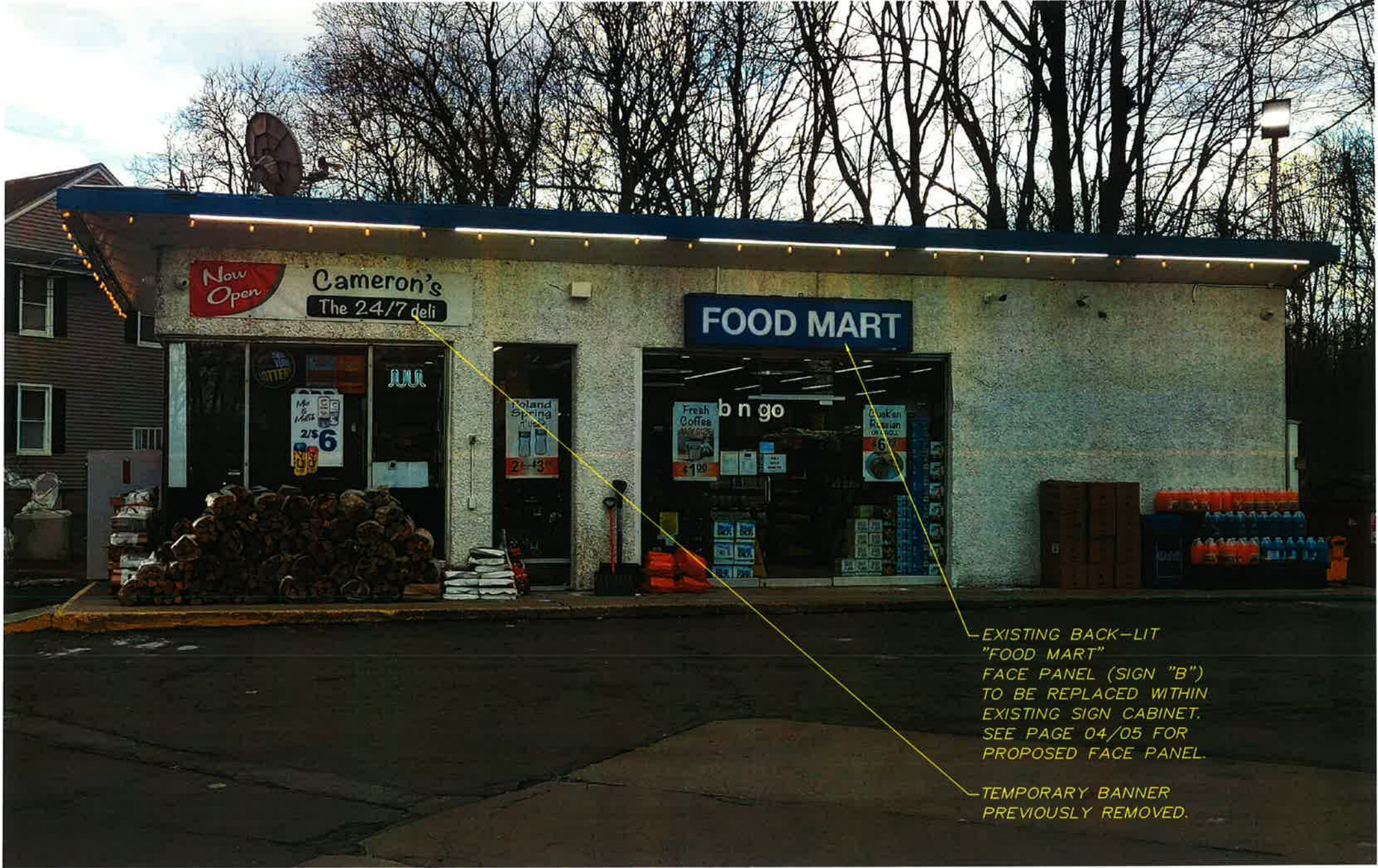
BUILDING FACADE WITH EXISTING SIGNAGE
